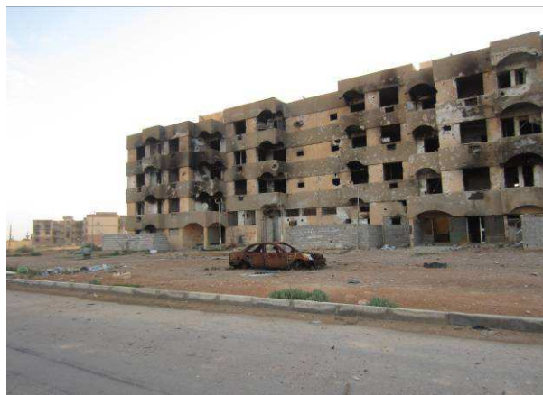
A deserted apartment building in Tawargha, burnt and pitted with small arms impacts, February 2012 © Amnesty International
