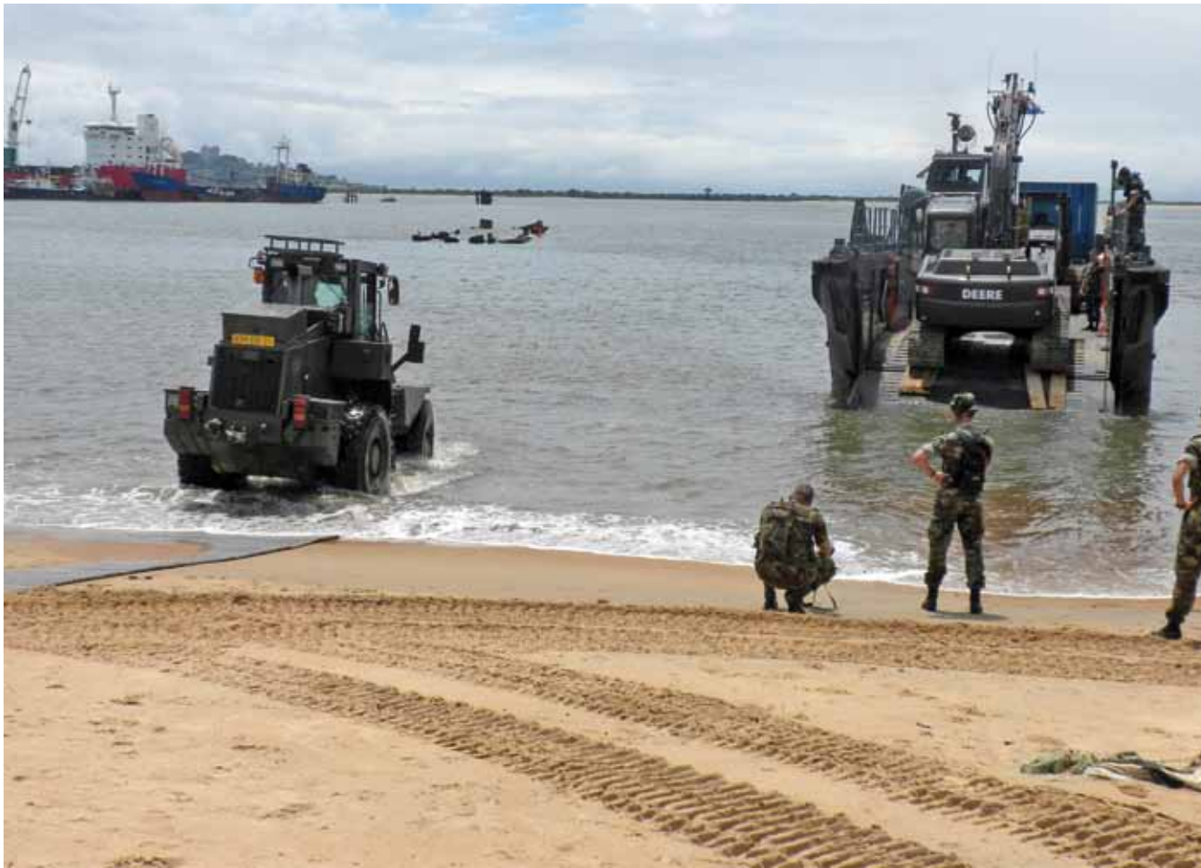
REBUILDING LIBERIA COAST GUARD BASE (above) - U.S. Navy personnel and equipment from Naval Mobile Construction Battalion Three in Rota, Spain, are transported to shore in Monrovia, Liberia by amphibious landing craft attached to the Dutch Africa Partnership Station platform HNLMS Johan de Witt (L 801), in October 2009. The Seabees were in Monrovia to rebuild the Liberian Coast Guard base that was destroyed in the country's civil war. (U.S. Marine Corps photo by Gunnery Sergeant Michael Maschmeier)
