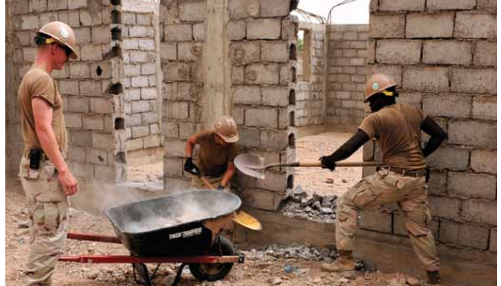
DJIBOUTI SCHOOL - Service members with Naval Mobile Construction Battalion (NMCB) 7 remove debris from Ecole 5, a five-classroom school in Djibouti on June 30, 2010. NMCB-7 is operating out of Camp Lemonnier, Djibouti. (U.S. Navy photo by Chief Petty Officer 2nd Class Nathan Laird)
